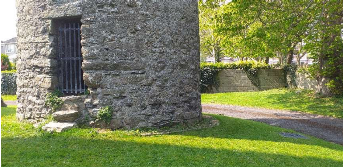
Base of tower with breezeblock concrete wall behind
