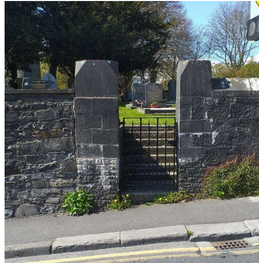
Pedestrian gate on Church Road
