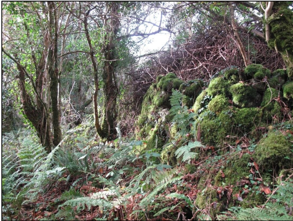
Plate 4: Wall at corner to south-east of site.
