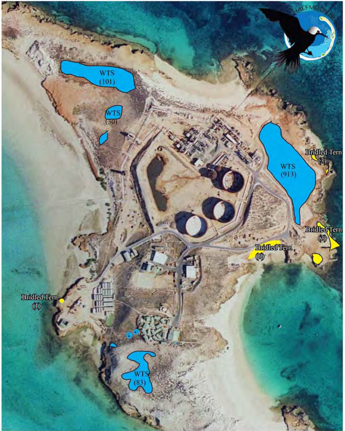
Figure 1: Aerial view of the Varanus Island showing the main seabird nesting areas located adjacent to proposed to Facilities Upgrades. Of note are the two Wedge-tailed Shearwater (WTS) burrows (see Figure 2) within the Kitchen Mess Cyclone Refuge (KMCR) area, and the single Bridled Tern nest site at the West Wharf. The WTS colony to the south of the KMCR site is approximately 40 m from the KMCR. Wedge-tailed Shearwater nesting burrows or habitat are shown in blue, and Bridled Tern habitat in yellow. The total numbers of nests/burrows Apache Energy Drawn by: C. Surman Date: 21 September 2012
