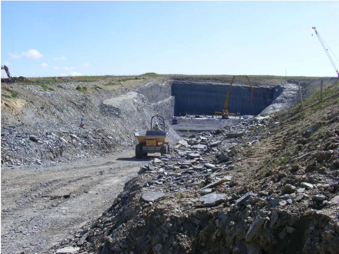
Figure 5.1: August 2012 – installation of the floor slab.
