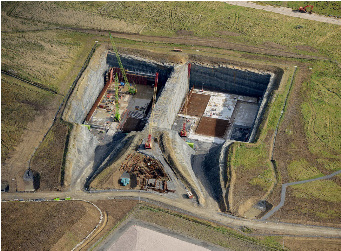
Figure 5.3: October 2012 – aerial view of construction.
