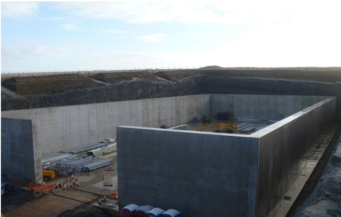
Figure 5.4: February 2013 – construction of reinforced walls complete.
