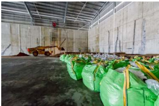
Figure 6.4: Photographs of Demolition LLW packaged in 1 te bags (left) and the interior of the Demolition LLW vault in 2017 showing emplaced layers of 1 te bags backfilled with sand (right).
