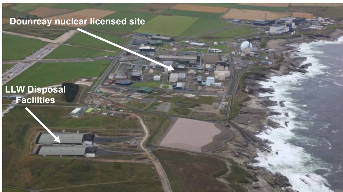
Figure 1.1: Aerial view of the Dounreay site in 2015 with the LLW Disposal Facilities in the foreground.
