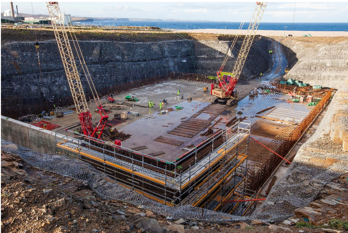
Figure 5.2: November 2012 – construction of reinforced walls.
