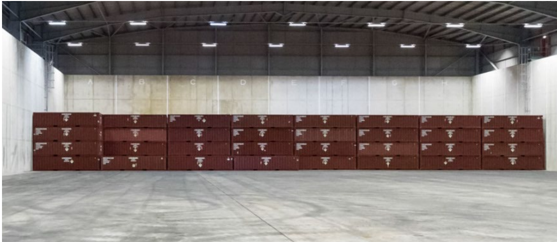
Figure 6.3: Photograph from 2018 inside the LLW vault showing emplaced HHISO containers stacked 4-high across the width of the vault.
