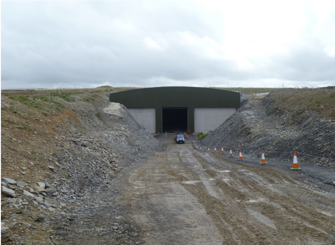
Figure 5.5: May 2013 – roof installation complete.
