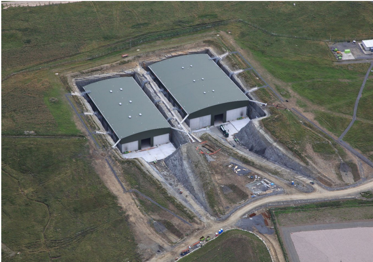
Figure 6.1: Photograph of the Dounreay LLW Disposal Facilities during construction (2012-2014).
