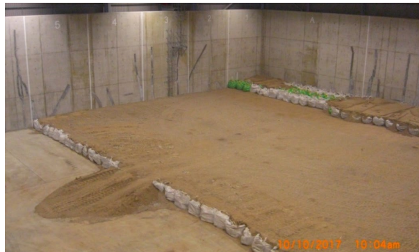
Figure 6.4: Photographs of Demolition LLW packaged in 1 te bags (left) and the interior of the Demolition LLW vault in 2017 showing emplaced layers of 1 te bags backfilled with sand (right).
