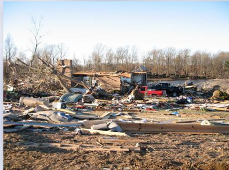
A home destroyed by a tornado in Jackson County, AL in 2008
