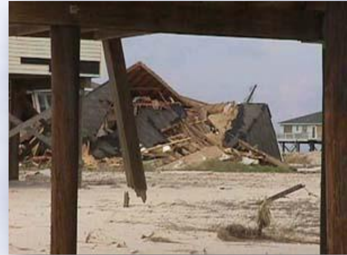
Homes destroyed on the Alabama coast by Hurricane Georges in 1998
