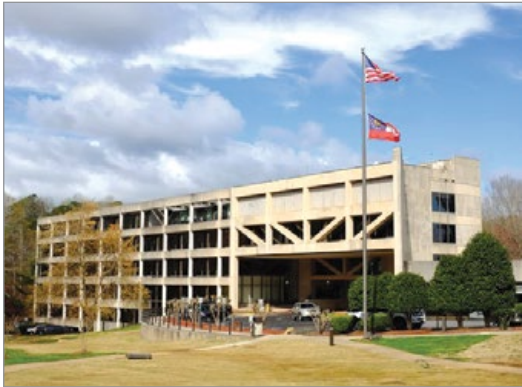
The Hall County Government Center has undergone a comprehensive energy and infrastructure upgrade through a collaboration with Trane.
