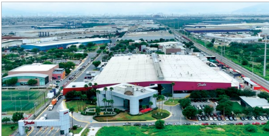
Mexico facility: Danfoss’ current facility in Apodaca, Mexico will be expanded with the construction of a new compressor manufacturing facility.
