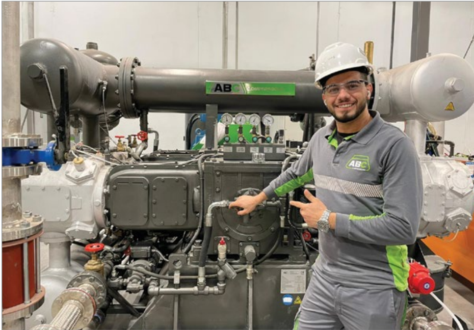
Start-up of an oil-free, reciprocating, high-pressure air compressor (photo courtesy ABC Compressors).
