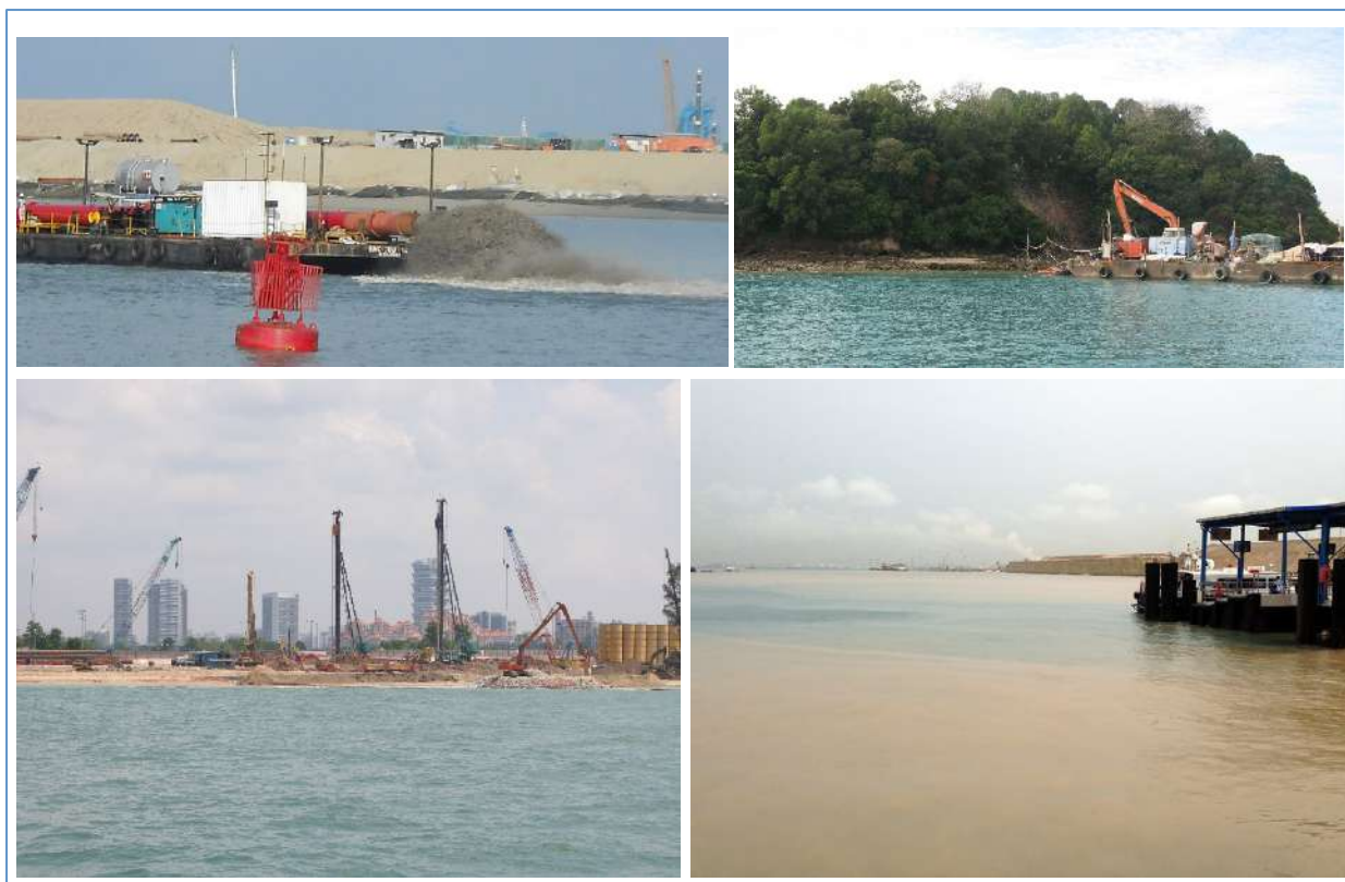
Figure 5.4. Coastal modification in Singapore (clockwise from top left): rainbowing of dredge spoil; slope mitigation at St. Johns' Island; significant sediment plumes occurring post rainfall during construction of Pasir Panjang Terminal Phase III; construction of Marina Barrage.
