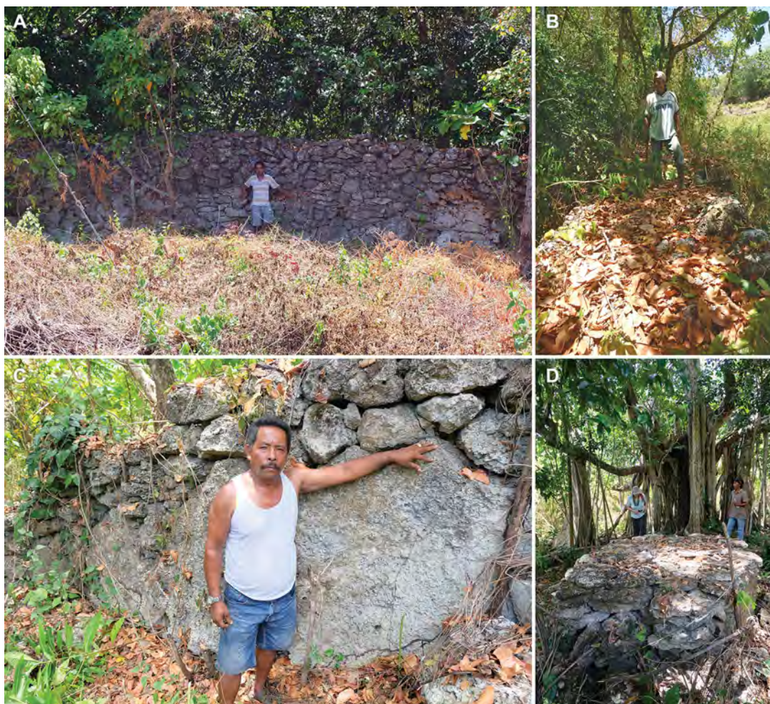
Figure 11.24. Kukeweble Negeri Lama (#61) showing the high (A), thick (B) surrounding wall constructed of a mix of medium to very large stones (C). In the centre of the Negeri Lama was a circular stone altar under the shade of a Banyan tree (D).
