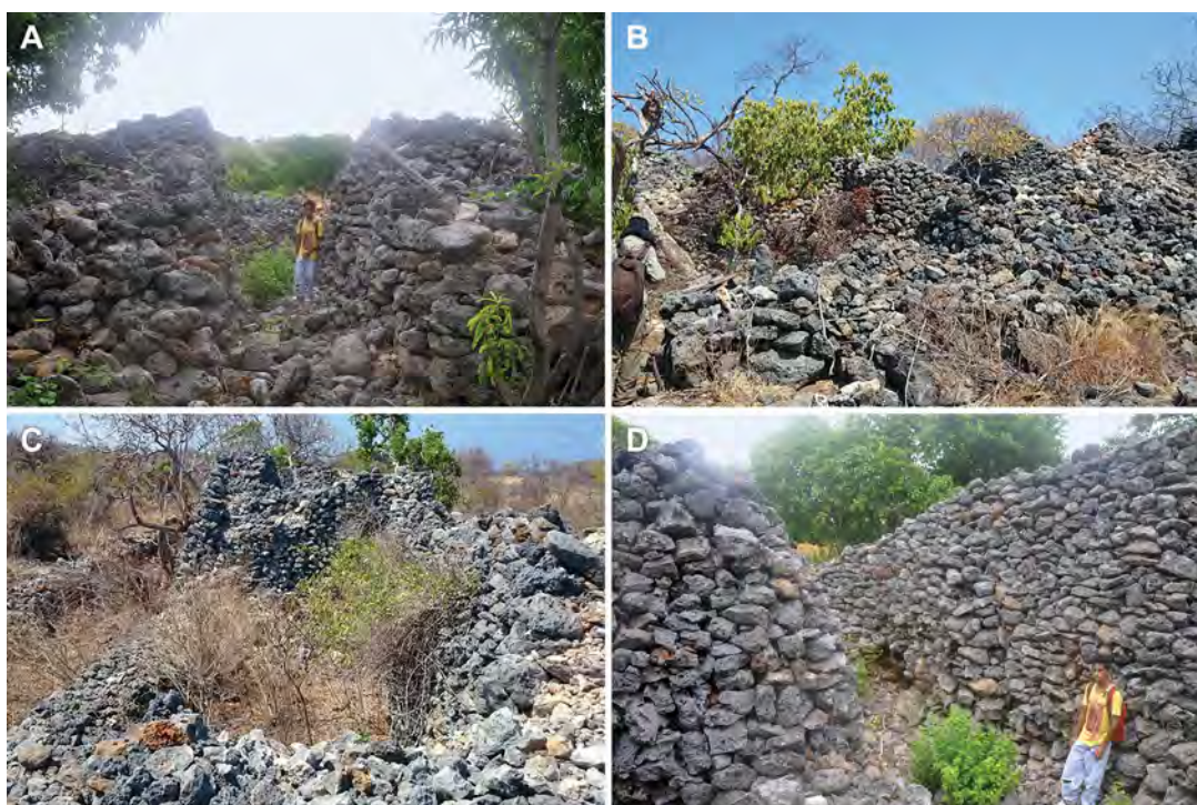
Figure 11.14. The Pur Pura Negeri Lama (KSR 49) showing the significant heights of the walls (A, D); extensive stonework (B) and chambers within the main wall dividing the headland (C).
