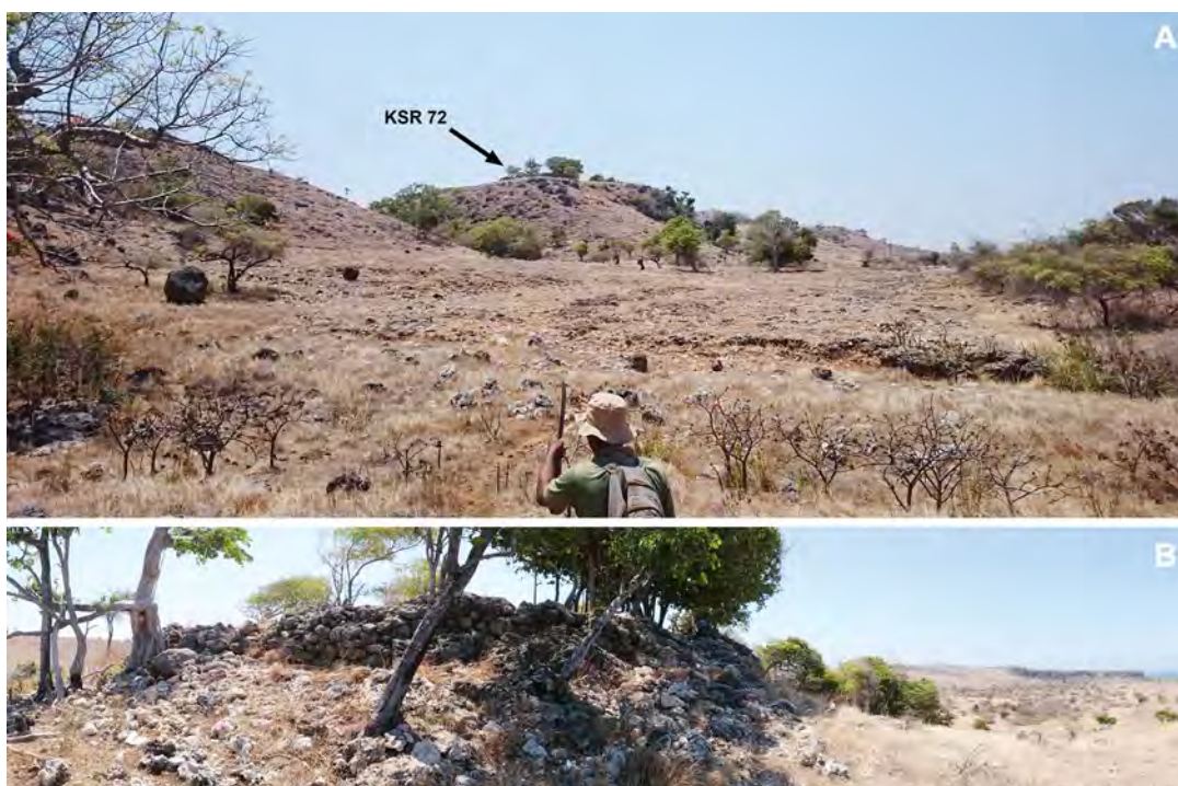
Figure 11.19. Nomaha Negeri Lama (KSR 72) view from plain looking north-northwest to the hilltop where the fortification is located (A), and the view of the stone wall looking north (B).
