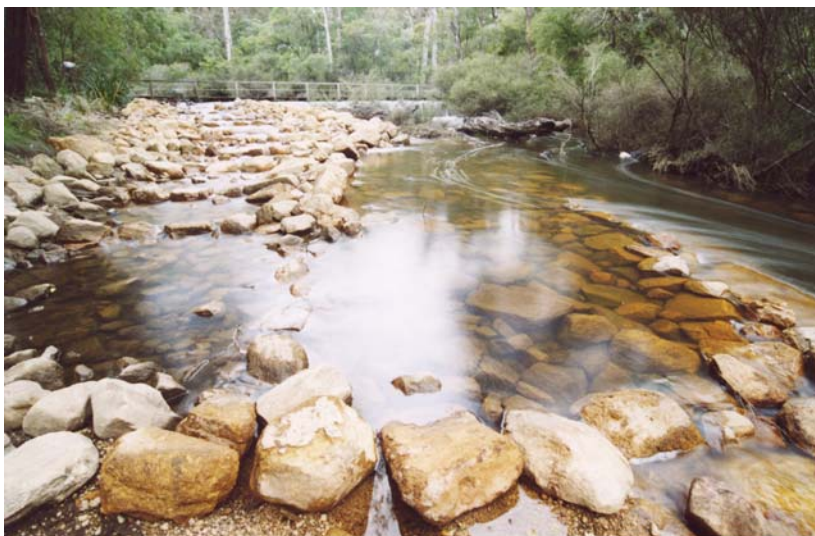
Plate 3 (Top) Goodga River vertical slot fishway, (middle) Hotham River rock-ramp fishway, and (bottom) Margaret River rock-ramp fishway (from Morgan and Beatty 2004a, b, c).
