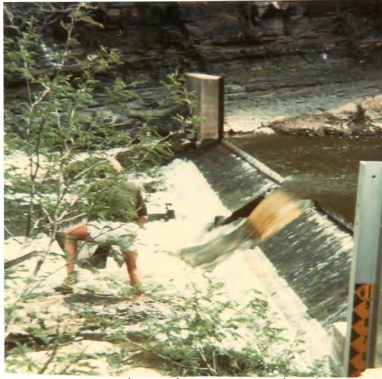
Figure 82 . Wolfcrag gauging weir on the Kowie River during "normal" low flow conditions.
