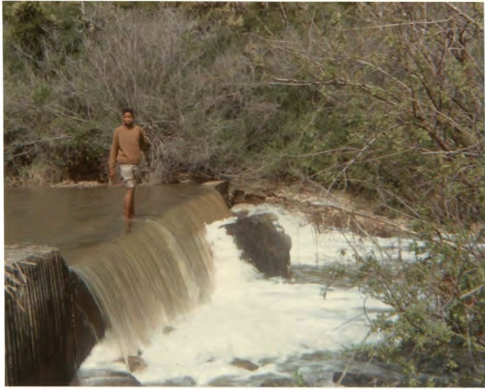
Figure 88. Weir on Kowie River ca 40 km from the head of the estuary, which prevents the upriver penetration of Myxus capensis . Note the water falls onto a shallow rock shelf below the wall.
