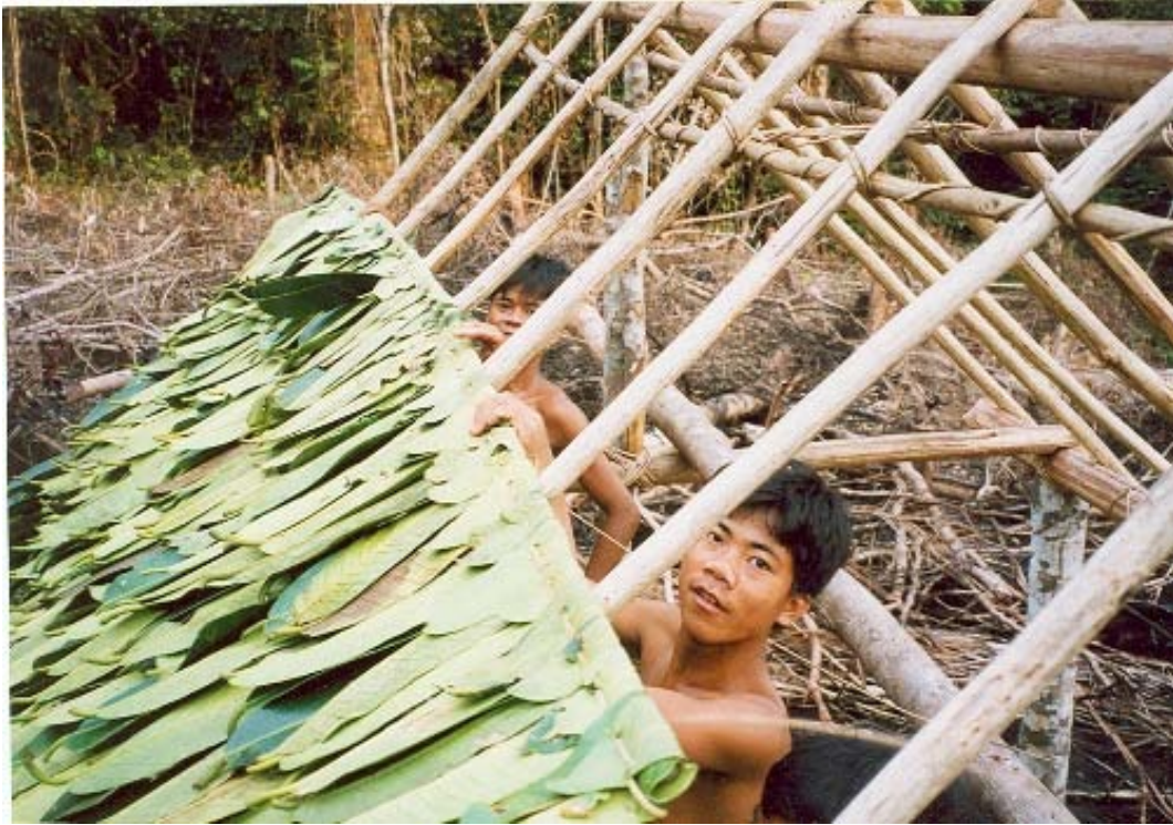
Attaching a Roof of Benal leaves
