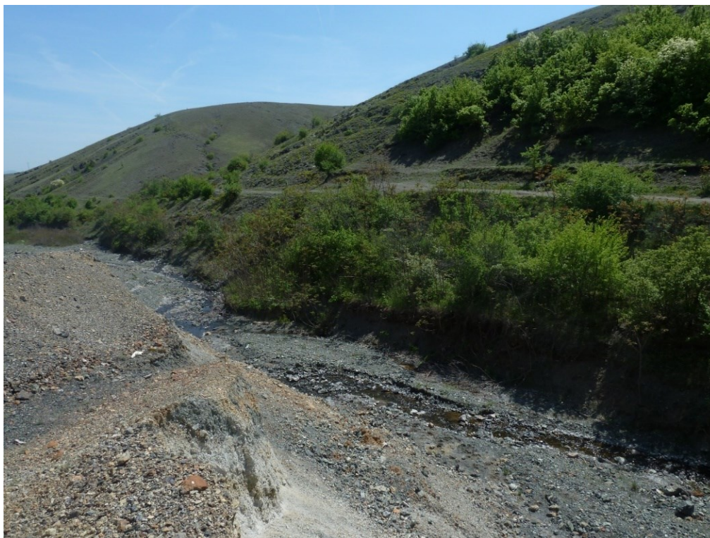
Fig. 3. Large ore-rich dump (left) whose western flank is eroded by the intermittently water-bearing small creek (right), Photo T. Đ. in April 2018
