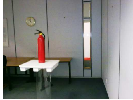
Figure 6.20 Fire extinguisher behind plywood wall
