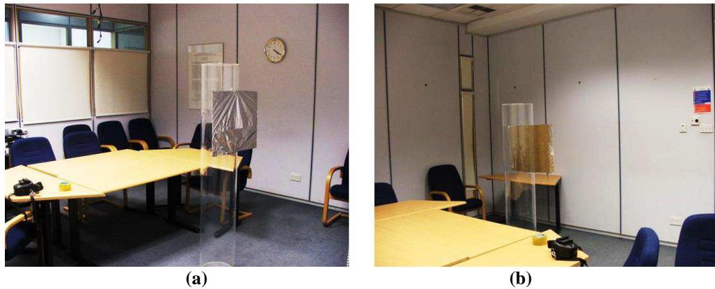
Figure 6.1 View of the scenario with plastered plywood wall: (a) the inside of the meeting room, and (b) the inside of the room with view of the plywood wall
