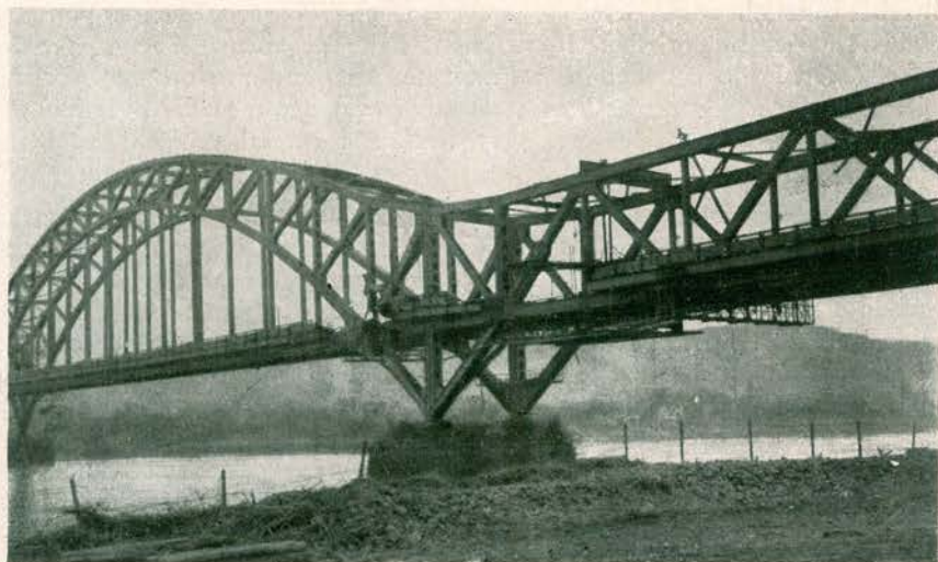
EAST END OF REMAGEN BRIDGE BEFORE COLLAPSE
