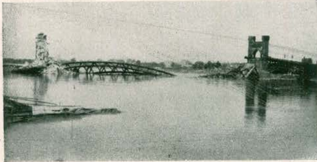
RHINE BRIDGE AFTER COLLAPSE
