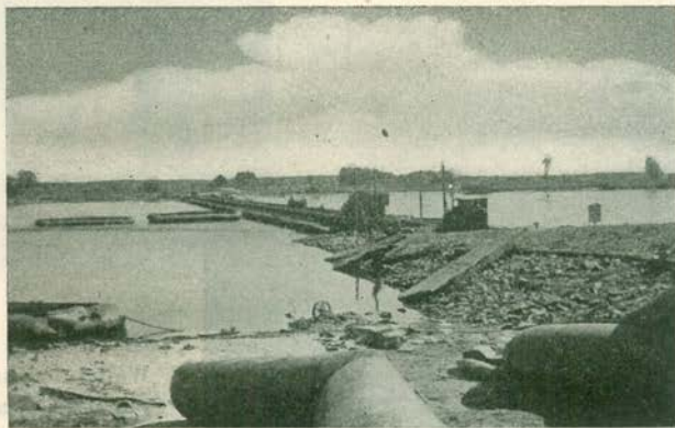
"By noon of April the 14th, NINTH Army Engineers had completed this treadway bridge."
