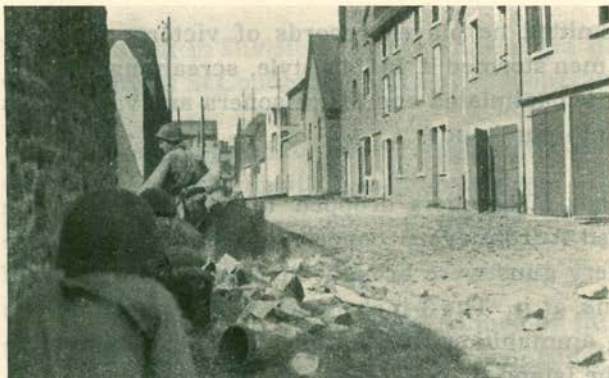
"A squad of riflemen proceed carefully down a street in St. Malo,"
