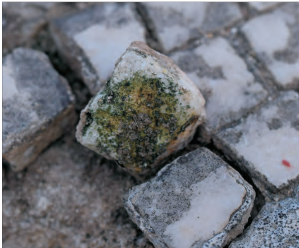
Fig. 2. Pigmented biofilm revealed below the mosaic tesserae in some area of the Leda's house peristyle .
