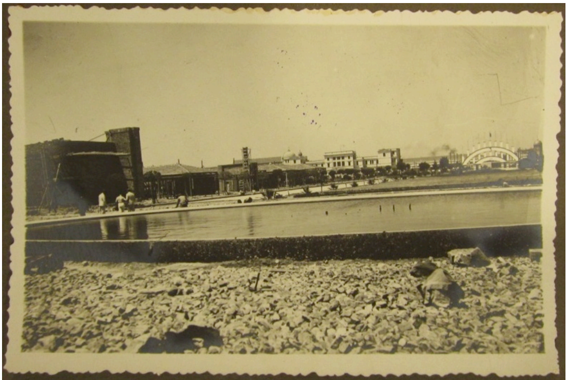
Figure 37. Photo taken inside Kültürpark , during construction. We can see the Greek Girls' School at the far back, and one of the gates of the park on the right. Sadi İplikçi Album, source: Mert Rüstem, İzmir.
