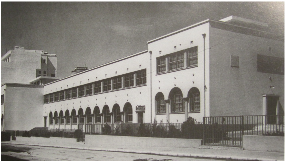
Figure 72. The Saint Sophia School complex, by Nikos Mitsakis, 1931. Source: Kolonas, Thessaloniki 1913-2013 , p.14
