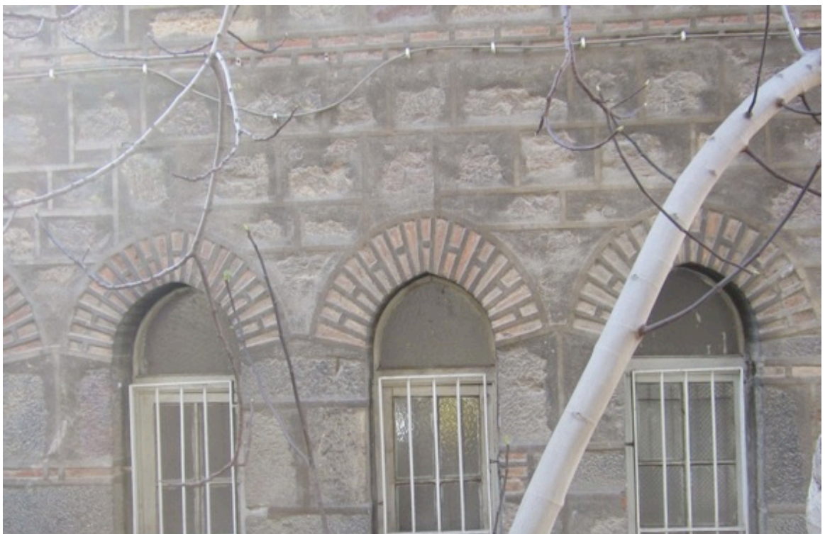
Figure 56. Windows on the northeastern facade. Photo by the author, 2013.
