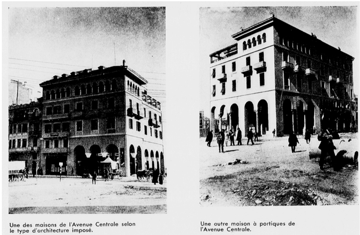
Figure 32. Buildings on today's Aristotelous Street, featuring the imposed facades. Source: Lavedan, 'L'Œuvre d'Ernest Hébrard en Grèce', p.161.
