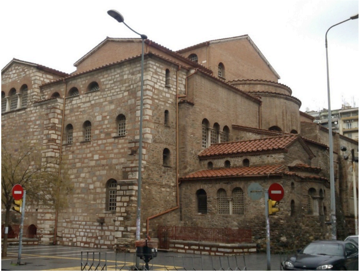
Figure 52. Photo (by the author) showing the connection between the old masonry and the one used by Zahos, 2014.
