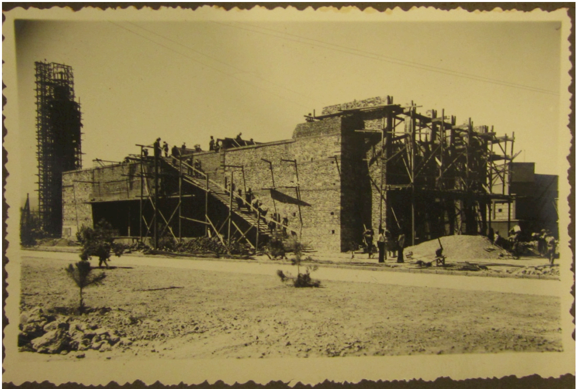
Figure 73. One of the pavilions in the International Fair. The Parachute tower can be seen under construction at the background. Sadi İplikçi Album, source: Mert Rüstem.
