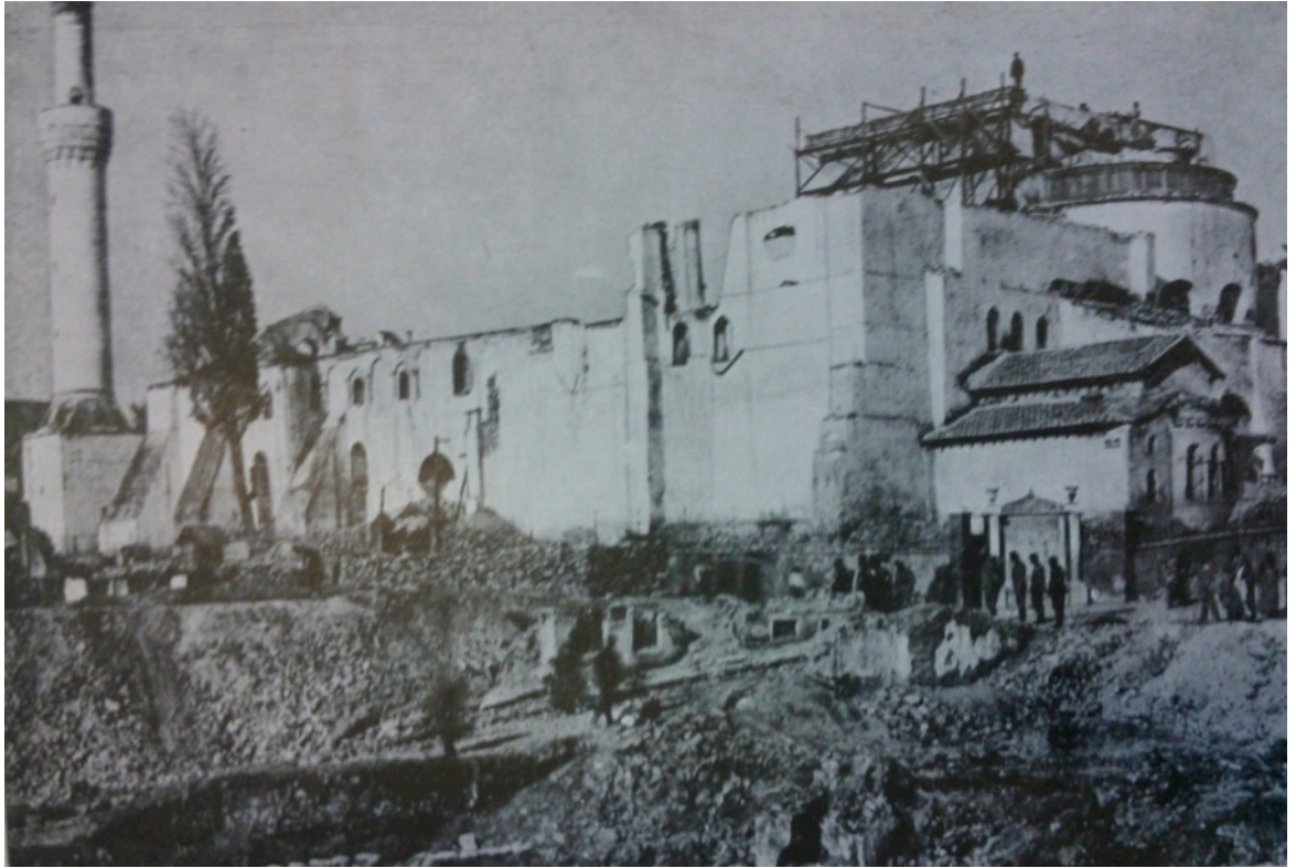
Figure 50. The church after the fire, exterior view with the minaret visible. Source: Sotiriou, I Vassiliki tou Agiou Dimitriou Thessalonikis , Photographic album accompanying the main publication.
