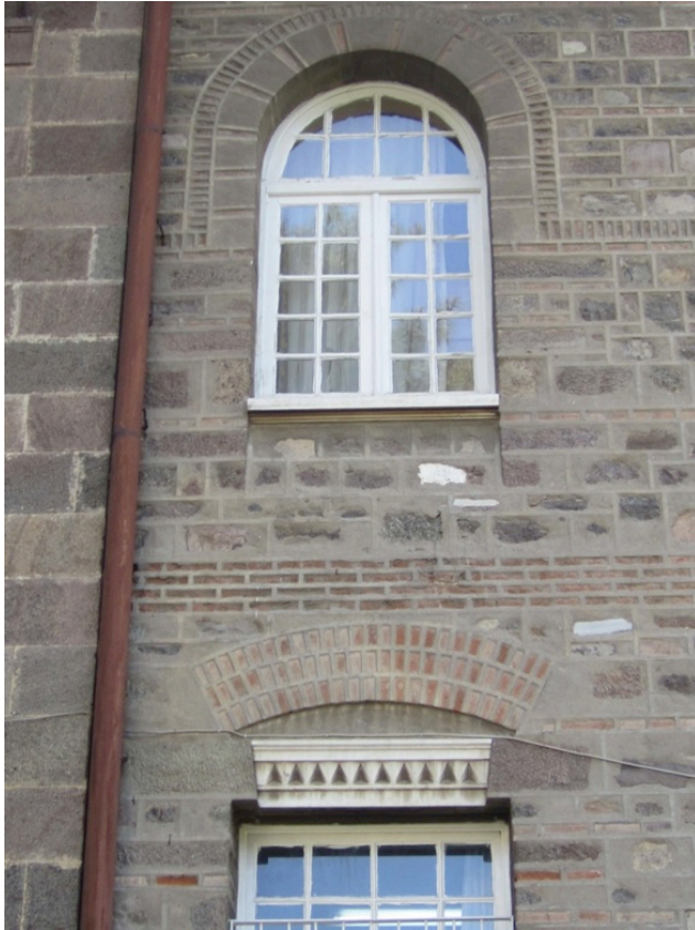
Figure 55. Detail of the front facade. Photo by the author, 2013.
