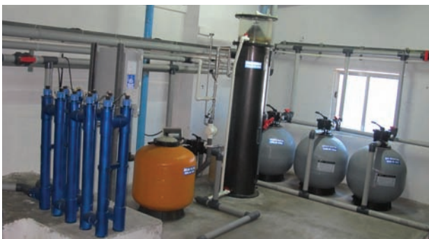
Indigenous RAS components (UV filter, Bead filter, Protein skimmer & Reactors)
