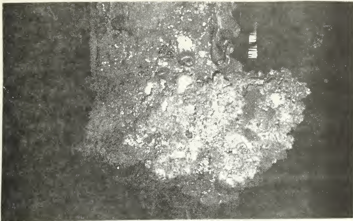
Figure 10. Biotic collar on a piling adjacent to Piling "B" extended from the low intertidal zone to shallow subtidal depths. Most of the mass is composed of Balanus nubilus shells.
