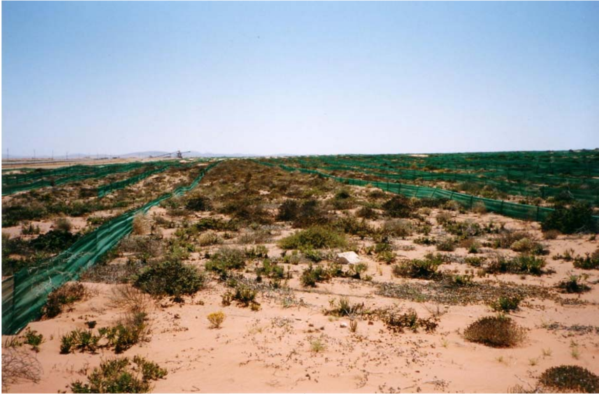
Plate 3.1: Windbreaks were erected perpendicular to the major wind direction in Site S1 in order to control wind erosion, prevent the loss of the soil's seed bank and prevent damage to plants.
