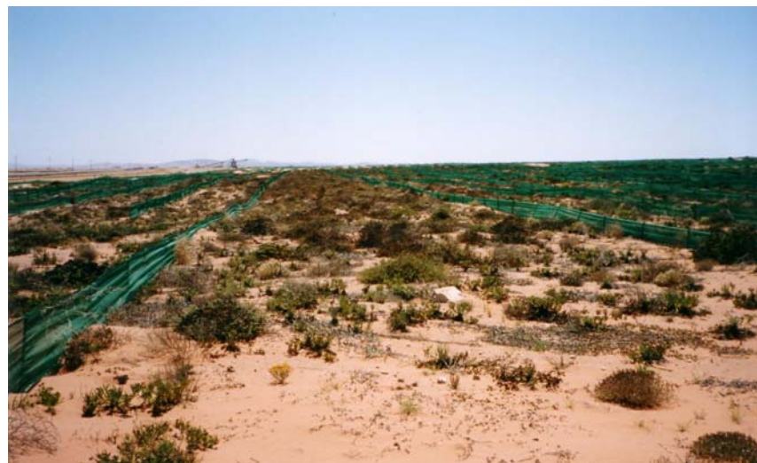
Plate 4.3: Rehabilitation site S1 was located in an area where topsoil was spread over tailings. Windbreaks were erected in all rehabilitation sites to control wind erosion.
