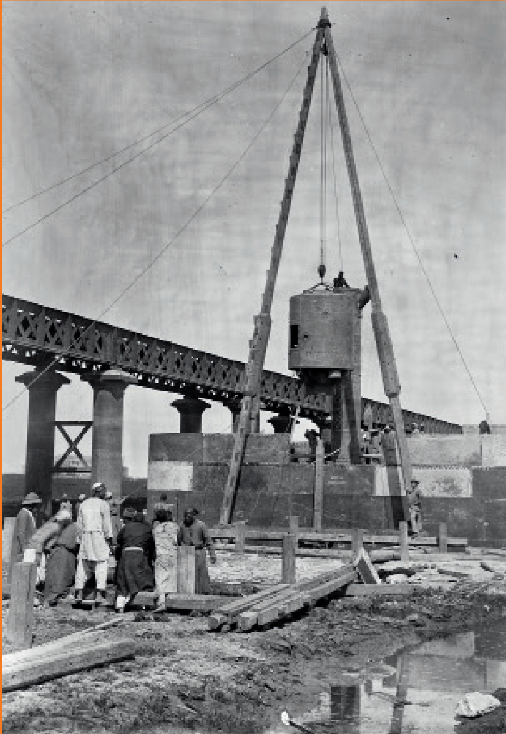
Kosheshah Bridge for the Egyptian State Railways, north of Beni Suef (1909): Sinking the pilings with compressed air
