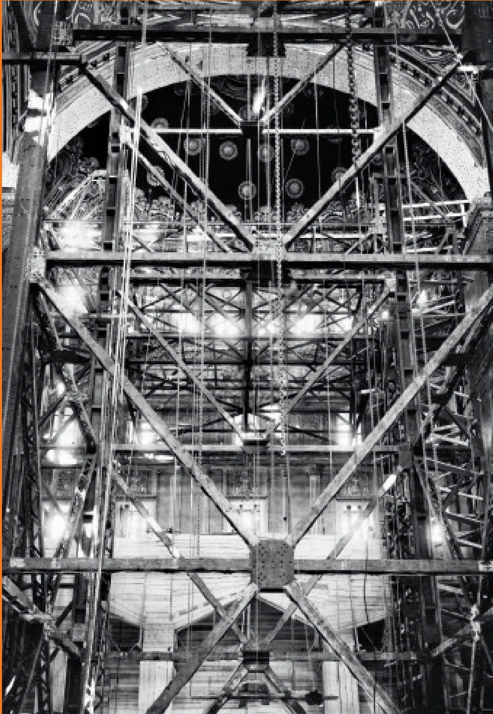
Muhammad Ali Mosque, Cairo: The interior scaffolding for restoration in the 1930s
