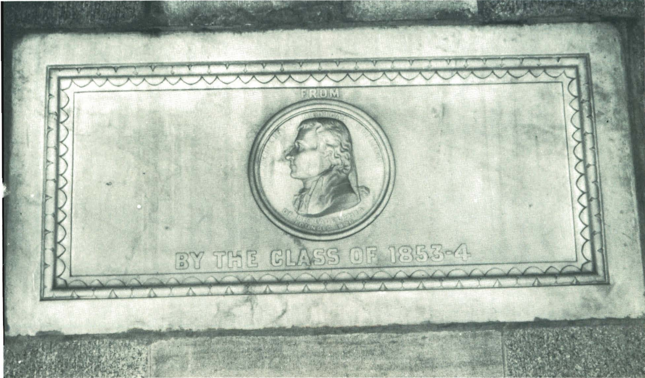
Fig. 55. Stone at 280-foot landing of Washington Monument, Washington, D.C. donated by graduating class of 1854. (Courtesy of U.S. Department of Interior, National Park Service.)
