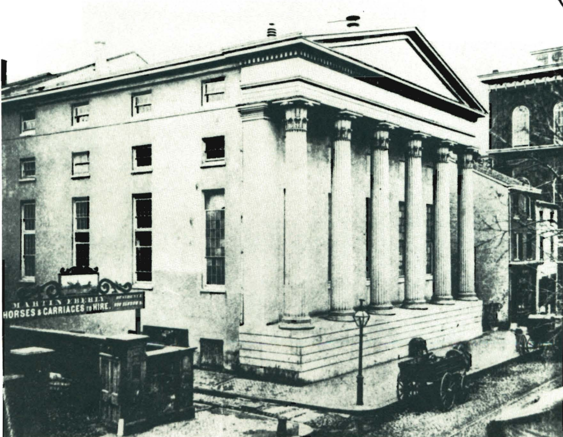
Fig. 39. The 1846 renovation of Medical Hall (Ely Building) with addition of a Grecian facade.
