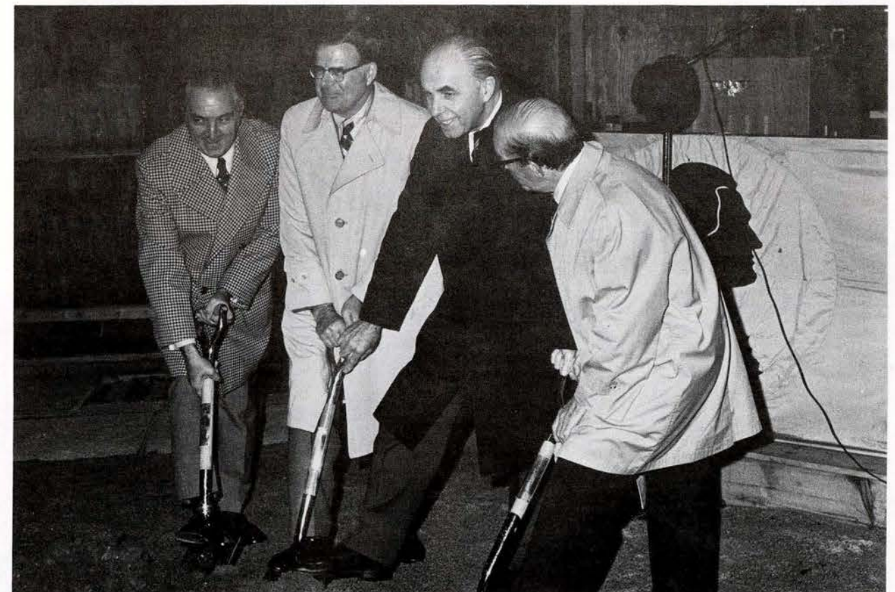
Mr. William W. Bodine, Jr., Chairman of the Board of Trustees of Thomas Jefferson University, and Dr. Peter A. Herbut, President, join with officials of the City of Philadelphia and the Hospitals Authority of Philadelphia in turning over the first soil at the ground-breaking ceremony on November 13, 1975.
