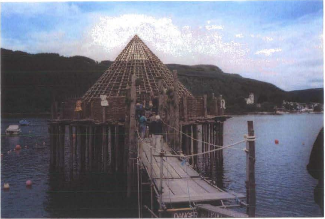
Fig. 4-29 Dixon's crannog reconstruction on Loch Tay, prior to thatching, summer 1996 (M.H.Davies)
