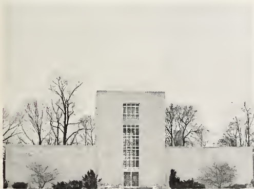
The modern Holcomb Observatory and Planetarium holds a 38-inch telescope. Tours of the building and planetarium shows are open to Butler students and the public.
