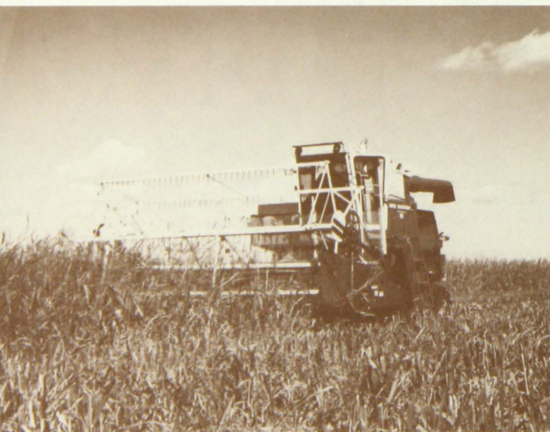
Figure 22. Harvesting wild rice with a modified rice combine.
