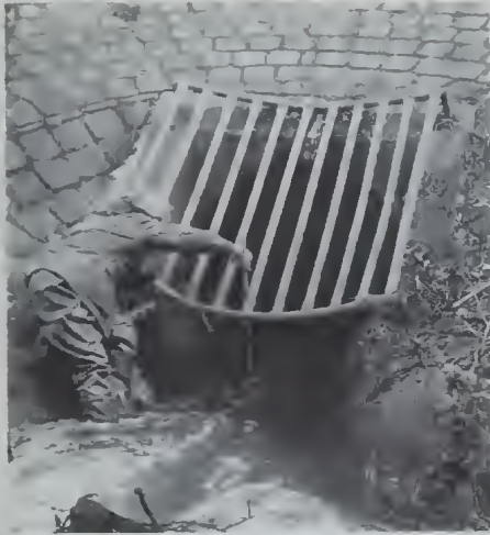
Fig. 1. Upstream end of the culvert conveying water from Monbulk Creek through the flood retarding basin embankment.
