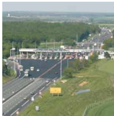
Opening of third lane to the north of Tours
