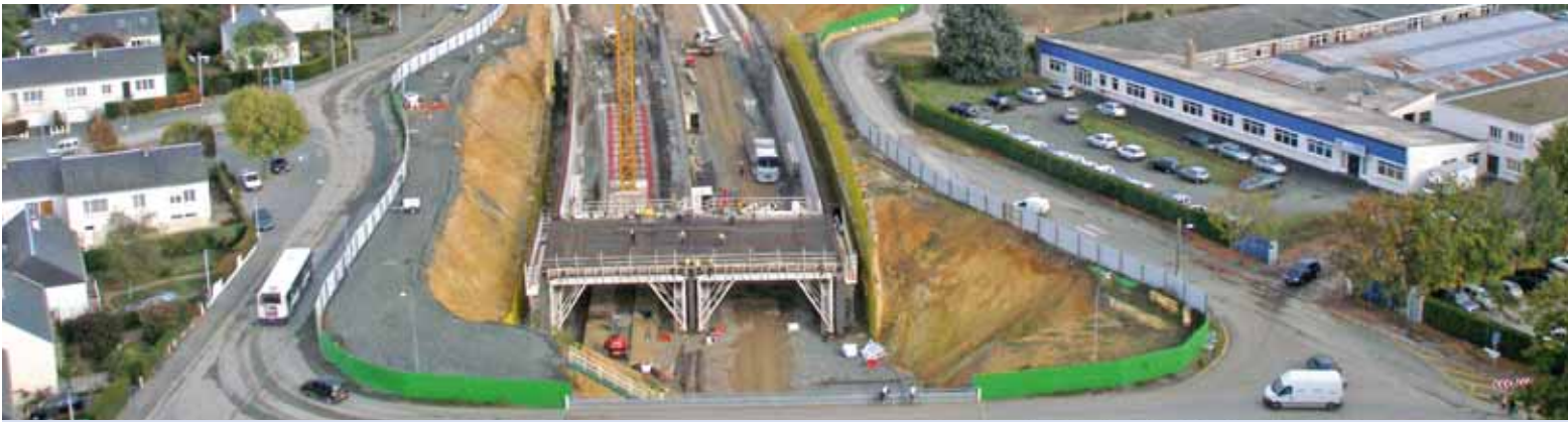
Construction of the cut and cover at Avrillé, A11 Angers
