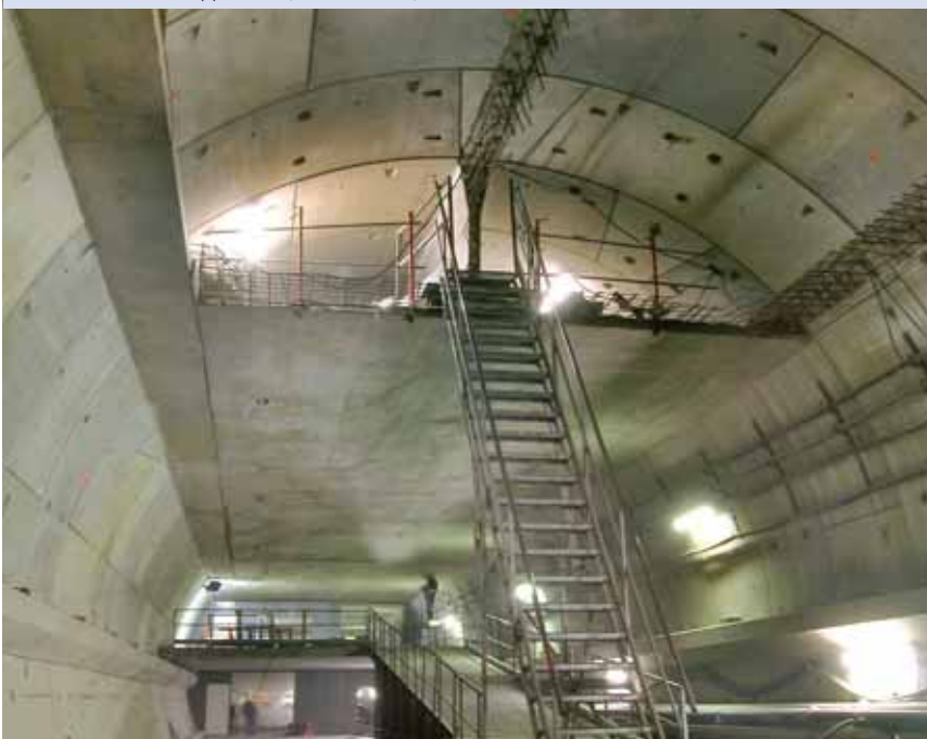
Construction of the upper slab (East 1 section)
