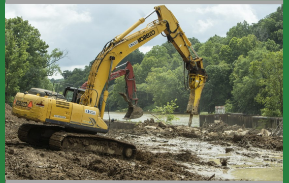
Photo: Equipment along the bank during dam demolition.
