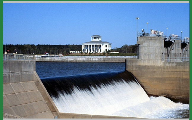
Photo: Tom Bevill Lock and Dam is one of the USACE lock and dam structures on the Tennessee-Tombigbee Waterway.
