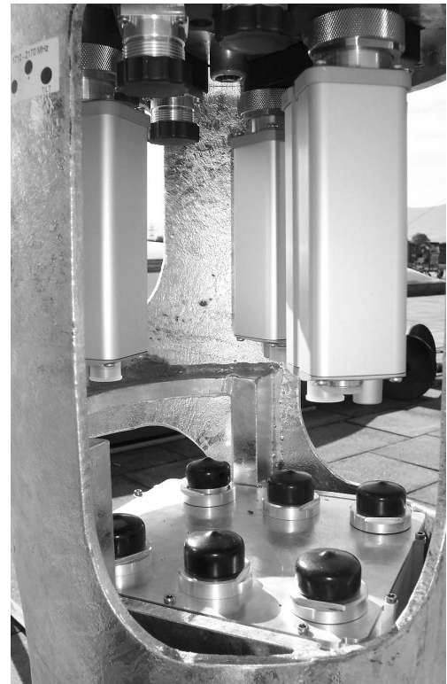
View inside service zone with MPTMA and Slimline RCUs
