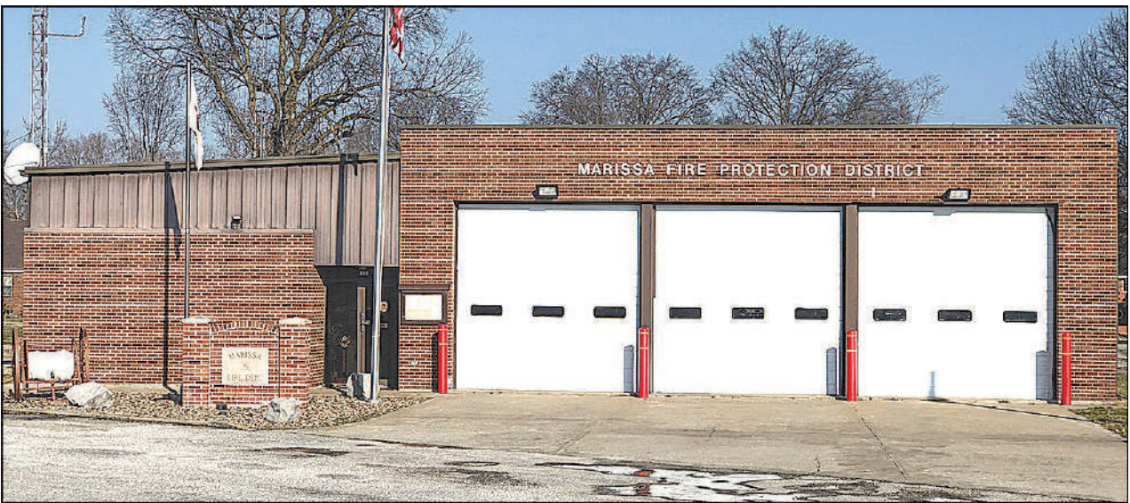
The Marissa fire station building will become the new home of the public works department.
