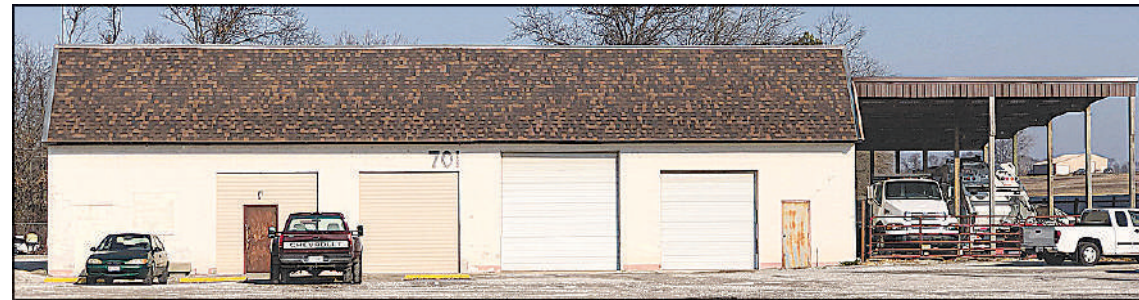
Marissa's public works garage will be the site of the new fire station.
