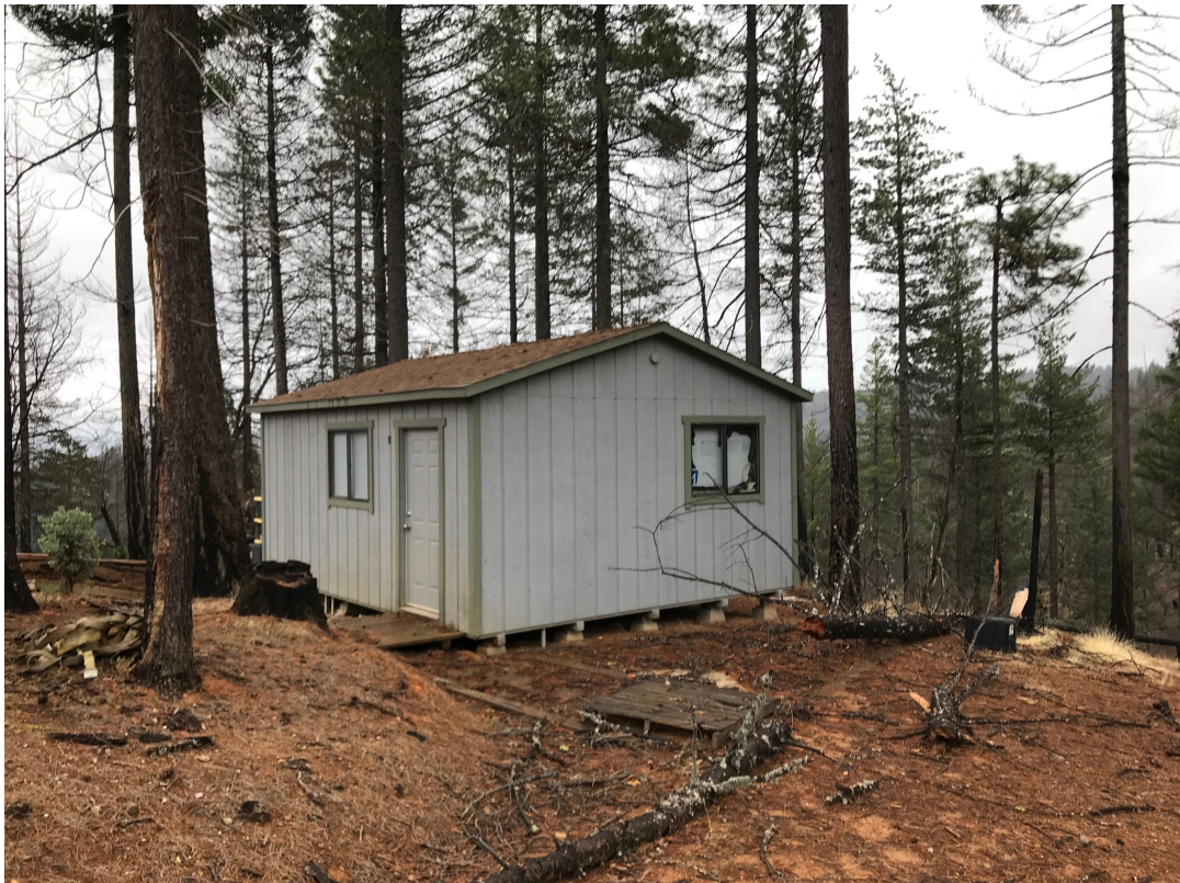
Existing Wooden Shed/Proposed Security Room/Building (east view)
