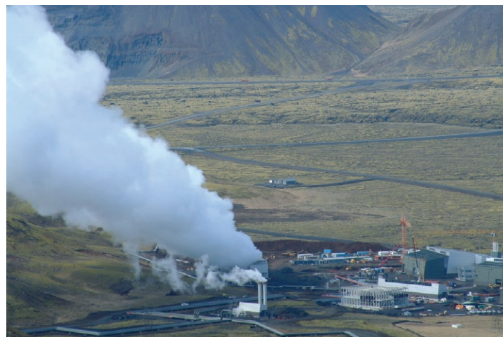
The CarbFix CO 2 injection site in southwest Iceland. The Hellisheidi power plant under construction is in the lower right, the moss-covered basaltic lava flow in the center of the figure, and the basaltic hyaloclastite (broken glass) mountains in the distance. The injection well is located in the lava fields in the upper left part of the photo. PHOTO: S. R. GÍSLASON
