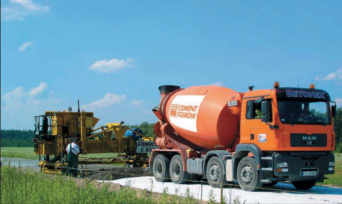
A section of a new six kilometre concrete road being laid by Grupa Ożarów for the town council in Ożarów. Concrete is seen increasingly as a cost-effective alternative for local roads in Poland.
