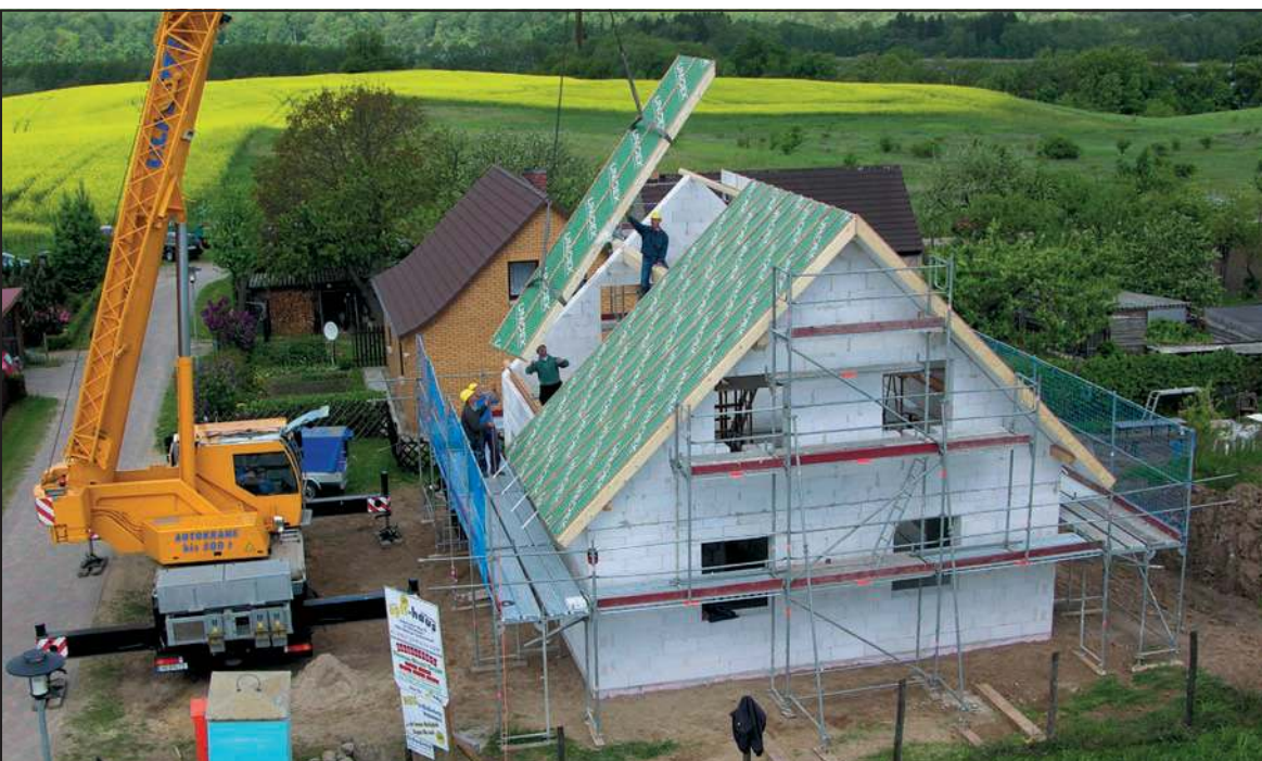
Uni-Plan Plus self-supporting insulation sandwich roofing elements are manufactured in the Netherlands by Unidek. Fitted on roof beams, these innovative elements remove the need for the traditional roof tile support system used in conventional pitched construction, reducing building time with considerable savings on building costs.
