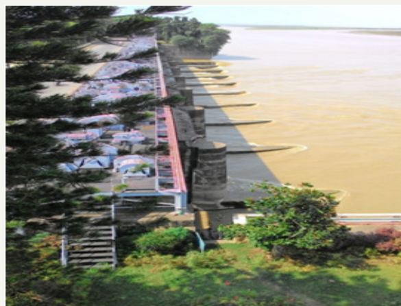
Figure 4c: The construction at the Feeder Canal head (Reproduced with permission from SANDRP).
