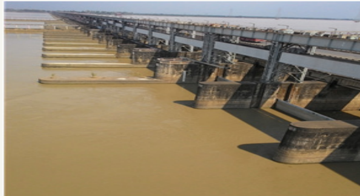
Figure 4a: Farakka Barrage (Courtesy of SANDRP).
