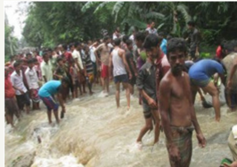
Figure 18 (c): People are repairing the broken dyke.
