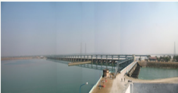
Figure 17 (b): Teesta Barrage at Gajaldoba with 54 gates that controls water discharge in Bangladesh.
