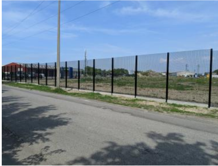
FIGURE 22: Author's photograph from 2019. Chemin du Pont-Trouille facing east after final eviction and installation of security fencing.
