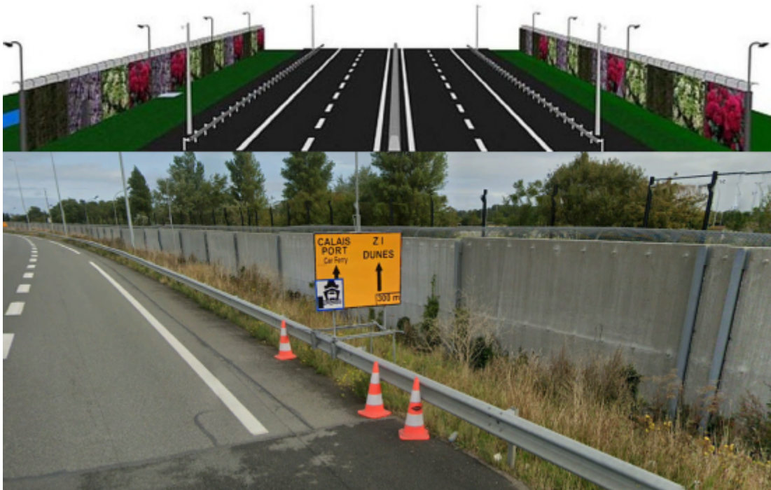
FIGURE 30: Composite of the architect's drawing for the 4m high 'Great Wall of Calais', with flowers and vegetation lining the interior, (top) compared to the actual wall (bottom). Images from Société d'Exploitation des Ports du Détroit, Port de Calais and Google Street View.
