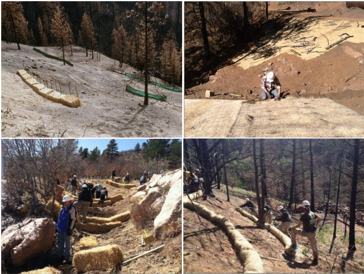
Figure 7-1. Examples of Emergency Stabilization Actions that BAER may Recommend.
