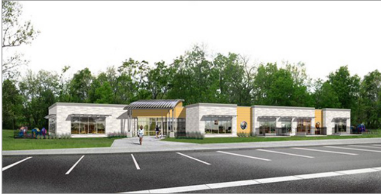
Childcare facility - LEED registered project
