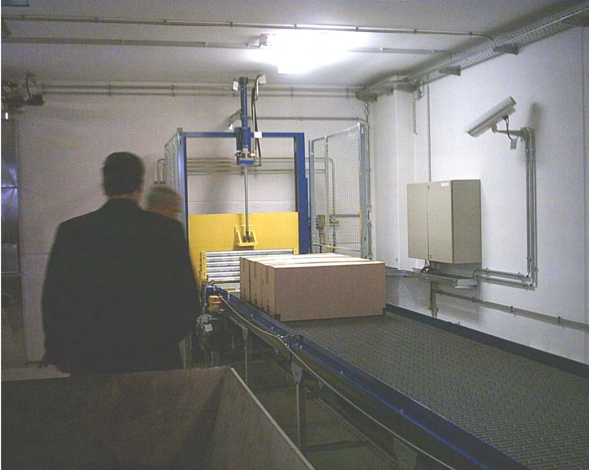
Figure 2-3: Inside of Loading Room, showing Feed Conveyor and Blast Isolation Door
