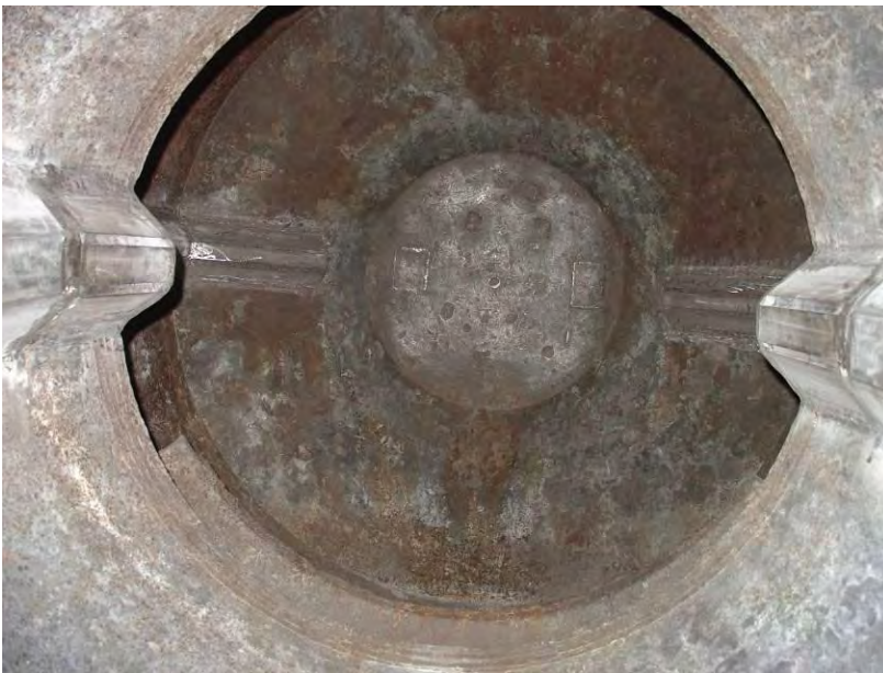
Figure 4-13: Inside of SDC 2000
