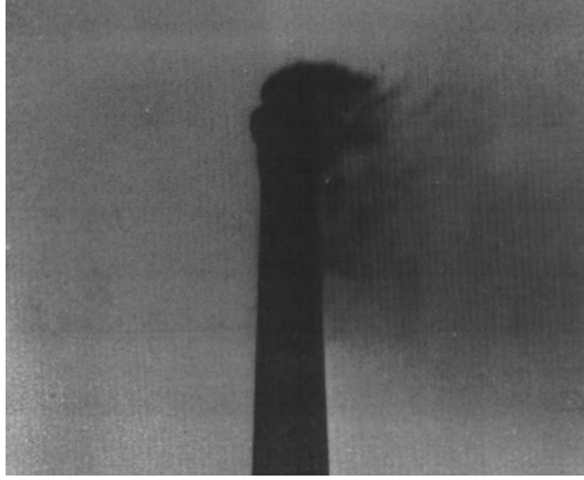
Figure 8-12. An example of downwash.
