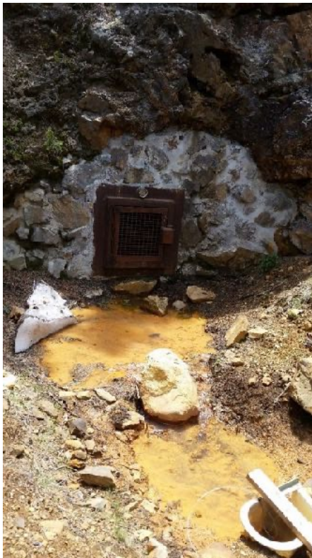
Buckskin Joe adit
