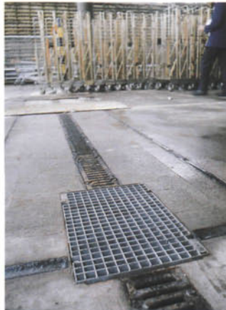
New modified drainage.
