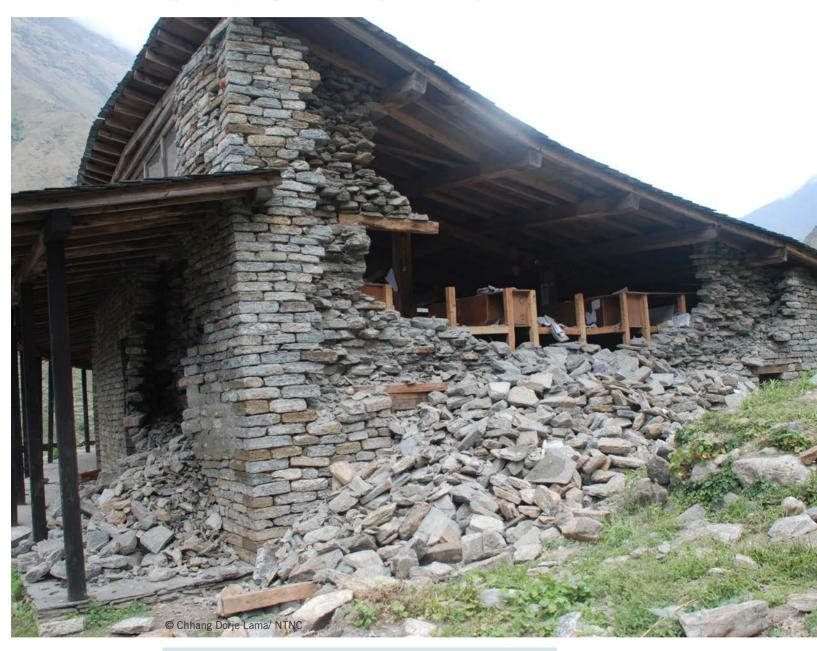
Photo 6: Damage caused by the earthquake in Buddha Secondary School, Gorkha
