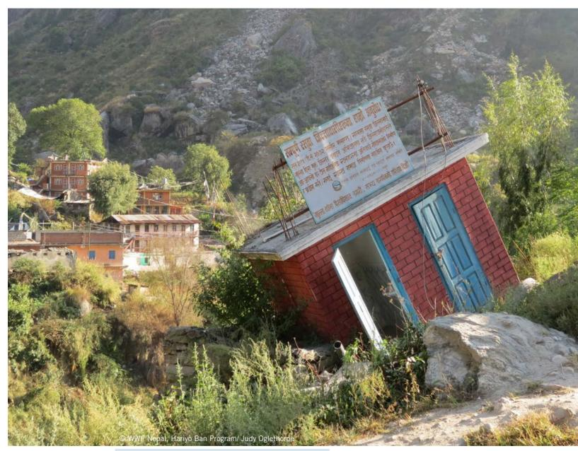
Photo 11: Public toilet damaged by the earthquake in Rasuwa
