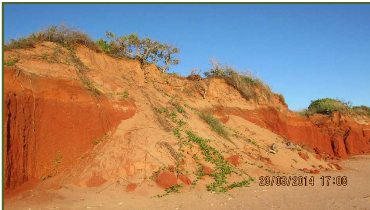
Pic 1.5 Corymbia paractia on eroding pindan at Reddell Beach.
