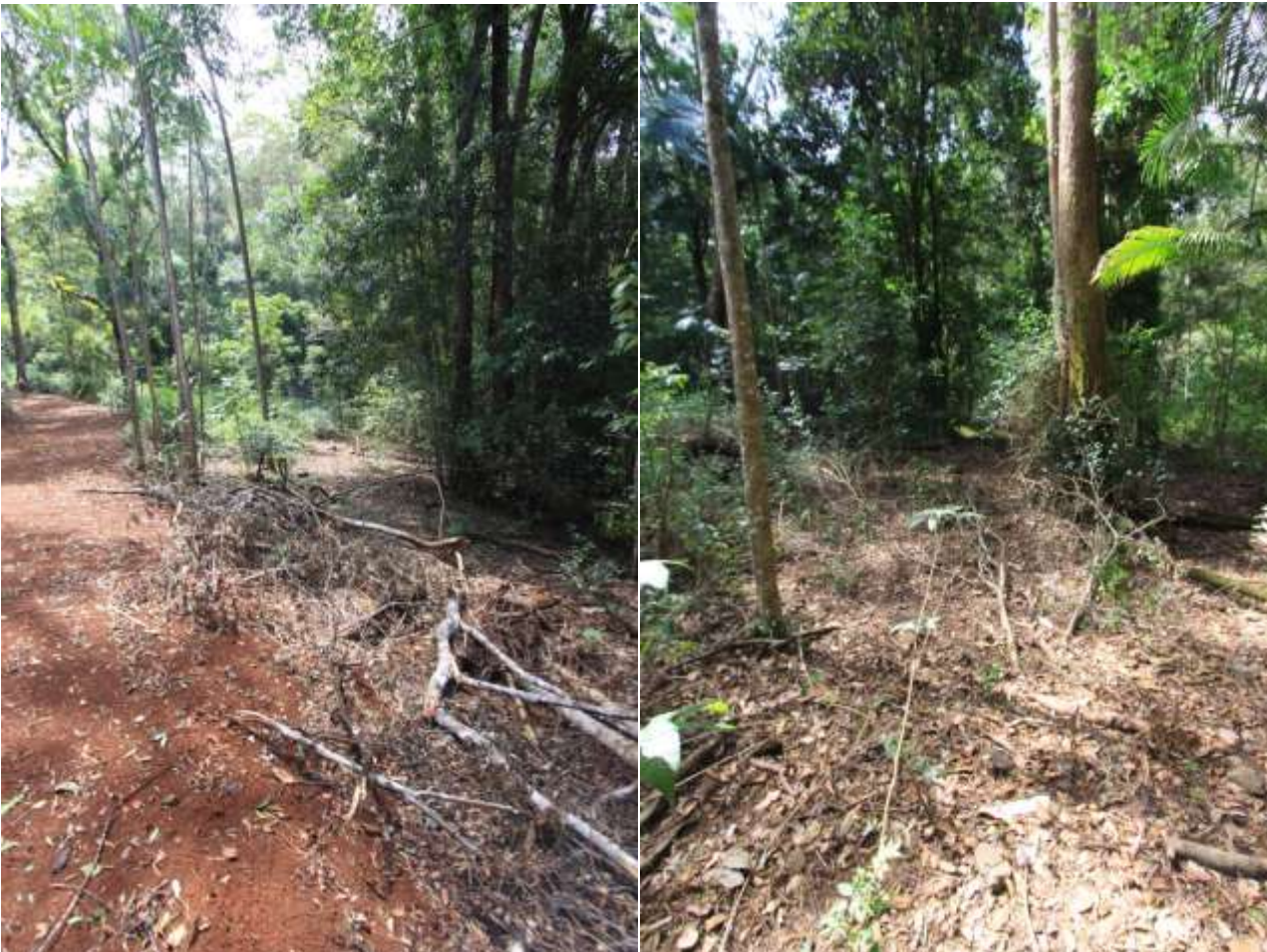
At two places within the rainforest bulldozer tracks headed off the main track, presumably the bulldozer was “going for a walk” to find a route for the road. See “side tracks” on map. TOP: (530312 6834390) extends for some 40m to south of road. BOTTOM (530098 6834490) extends for some 90m to north of road
