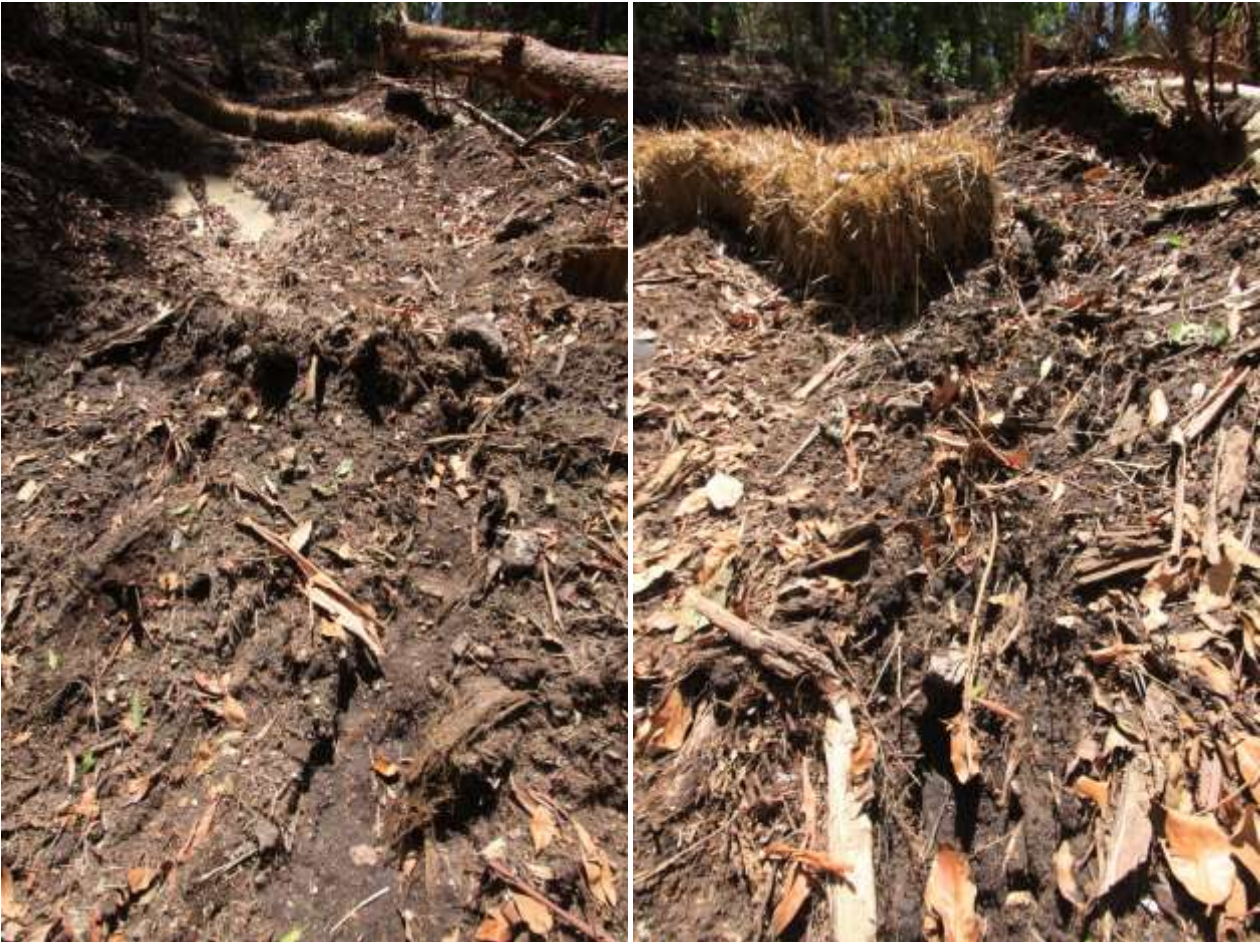
Failed cross-banks on extraction track.
