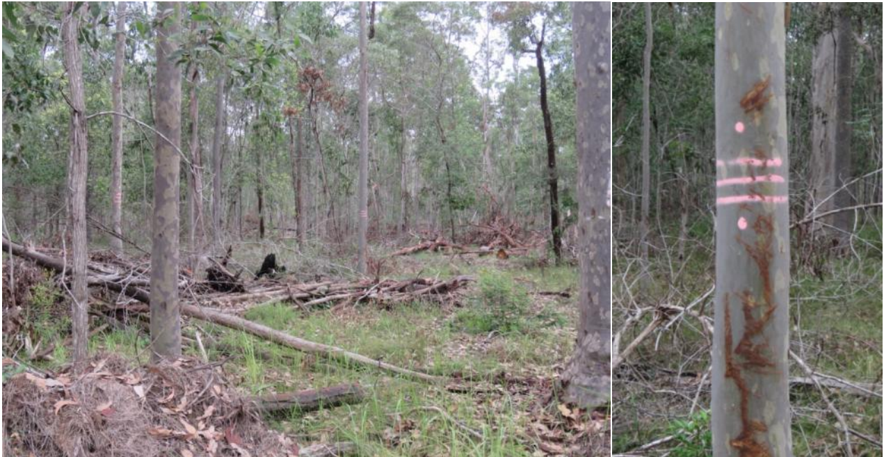
Logging into the boundary of the Melichrus exclusion area, with the boundary wrongly marked near the road with logging extending up to 44m from Melichrus. Note the appropriate boundary marking of "3 Machinery (3 bars 2 dots)",
