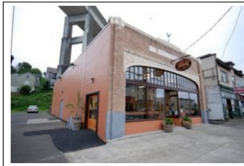
Figure 14.115-5: Non-Industrial Building, Flat Roof Behind Parapet Wall
