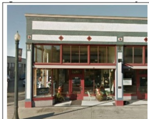
Figure 14.195-4: Prominent Main Entry
