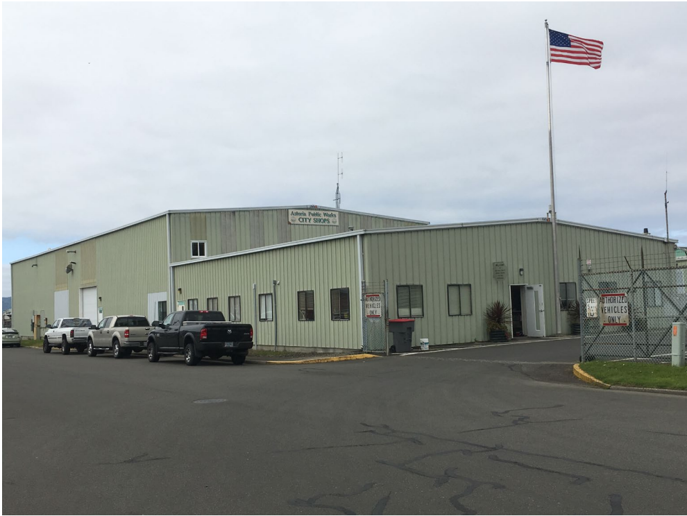
Public Works Shop – Looking North
