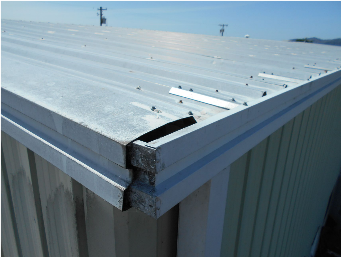
Roof (Upper Section) – Looking Northwest
