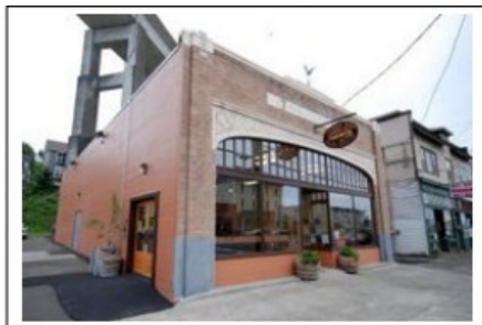
Figure 14.195-10: Non-Industrial Building, Flat Roof Behind Parapet Wall
