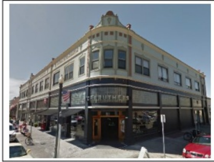
Figure 14.195-6: Corner Entrance and Features
