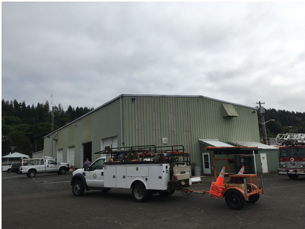
Public Works Shop – Looking South
