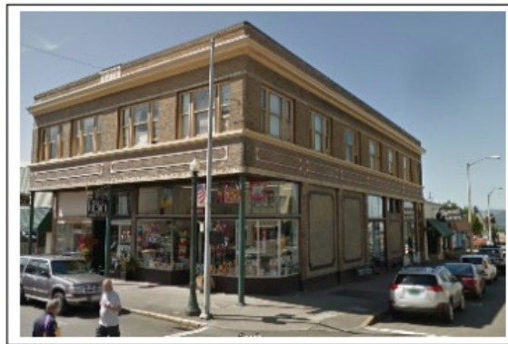
Figure 14.195-5: Base, Middle, & Top of Building
