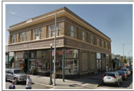
Figure 14.158-4: Base, Middle & Top of Building
