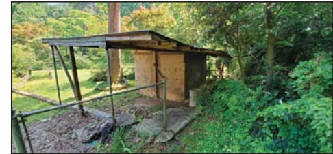
OLD GAZEBO BEING REMODELED
